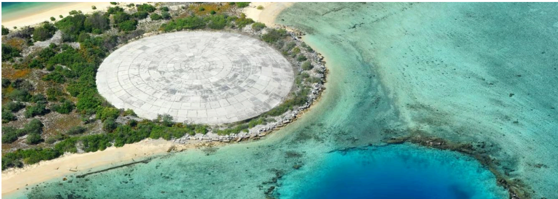
Figure 35 The Runit Dome
