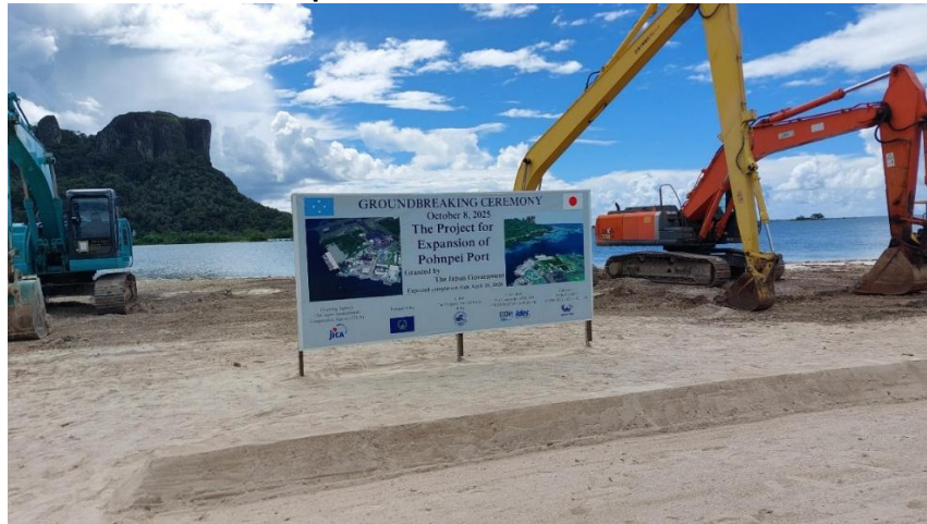
Photo 2: Planned Site for Port Expansion and Modernization on Dekehtik Island, Pohnpei
